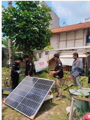
Gambar 5. Proses Perakitan Panel Surya
